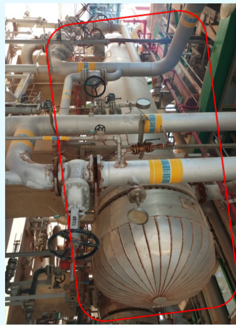
Figure 1. Oil-oil shell and tube heat exchanger
